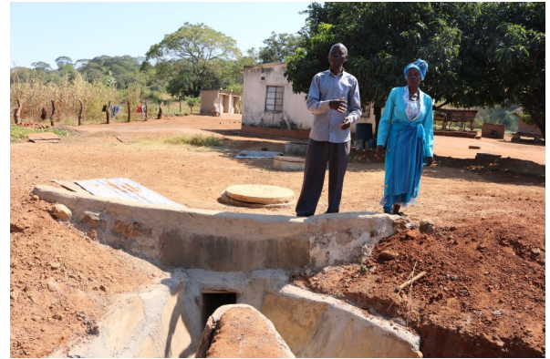
Image: Mr and Mrs Hlongwani explaining how the bio-digester works .
